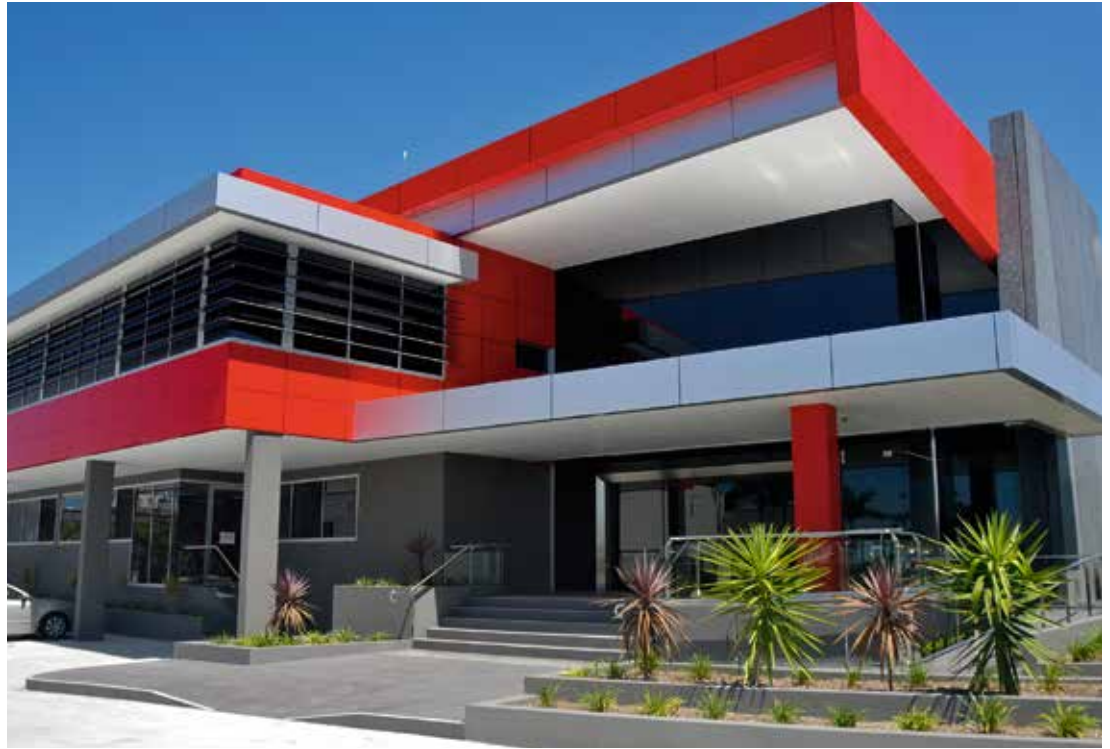
Innotech Controls Systems’ manufacturing headquarters.
