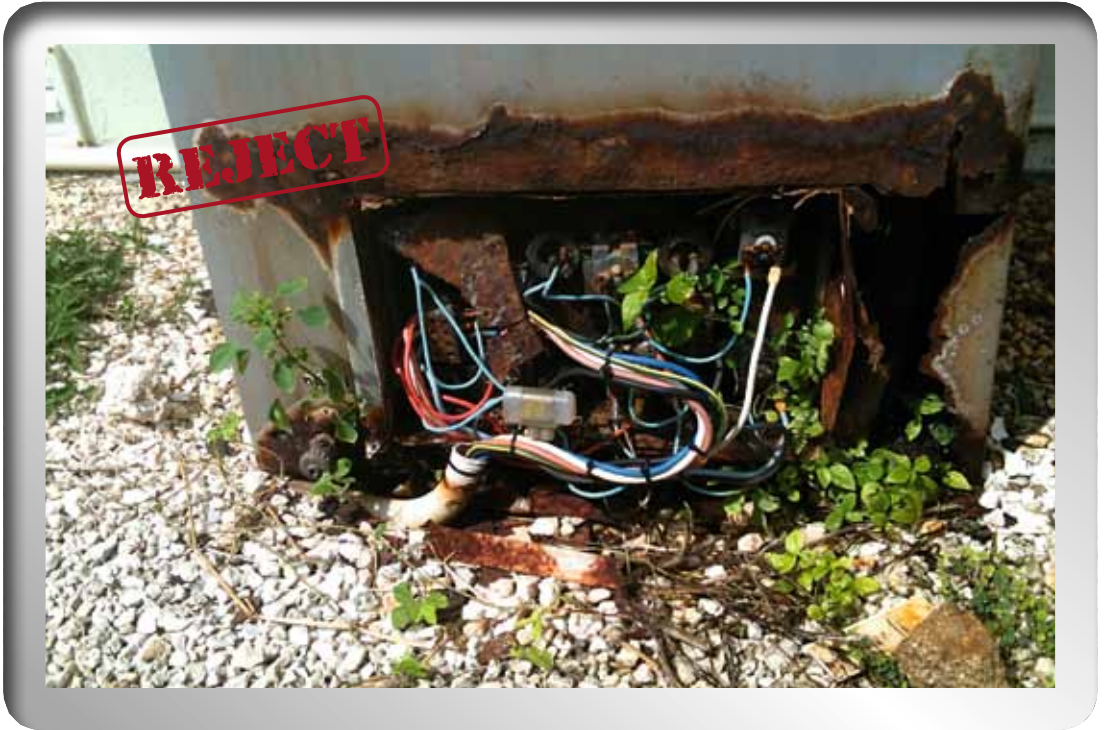
Exposed wiring.
