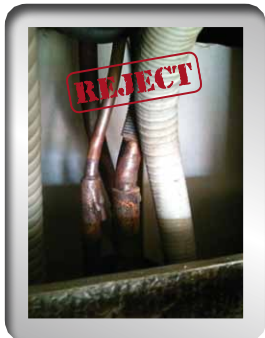
Different copper pipe sizing just slotted into each other and welded.
