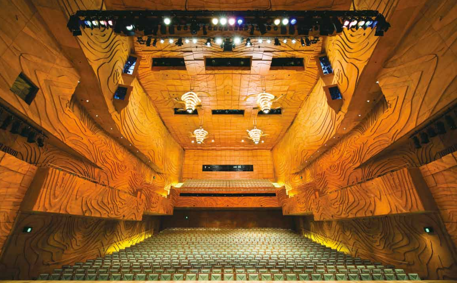
The Elisabeth Murdoch Hall sits within a cast-concrete box mounted on 38 spring assemblies, which isolates the building from the noise and vibrations of passing trams. Image: John Gollings.
