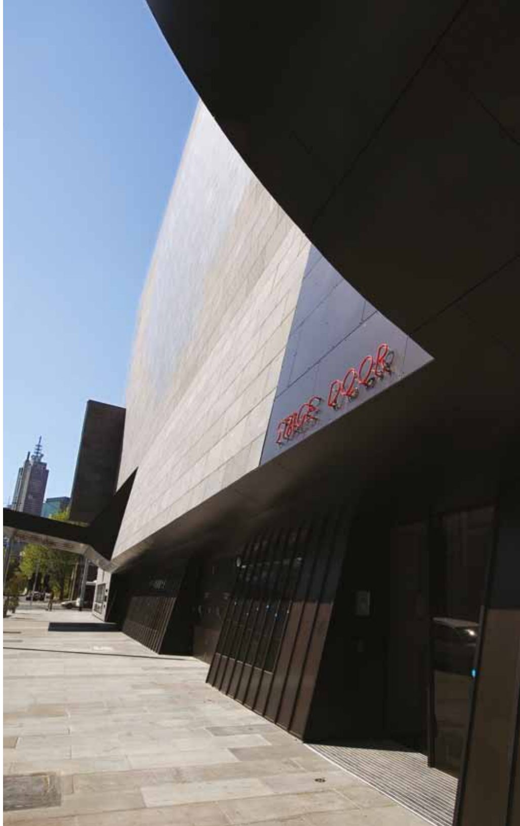
Controlling noise from external sources as well as patrons and buildings services was paramount to achieving the client's strict acoustic criteria.
