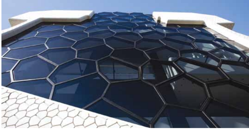
The glass panels on the external façade can open for natural ventilation.
